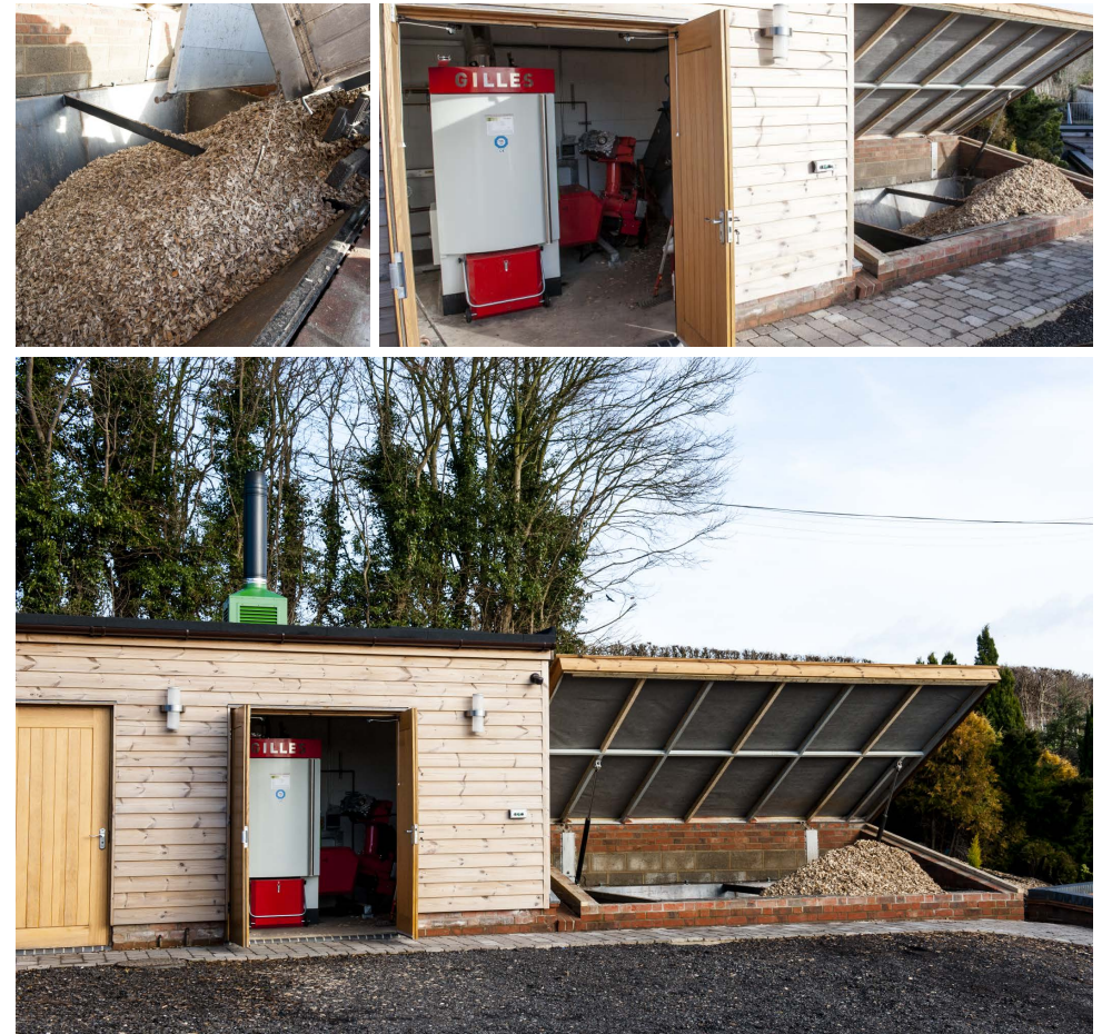
Domestic Biomass boiler running TMA Barks process dried woodchips.
